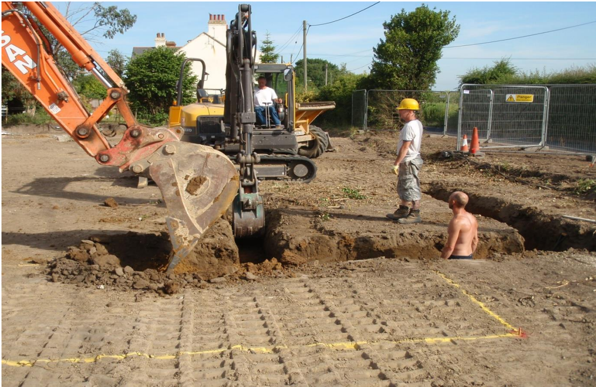
Plate 2. Cutting foundations Plot 7
