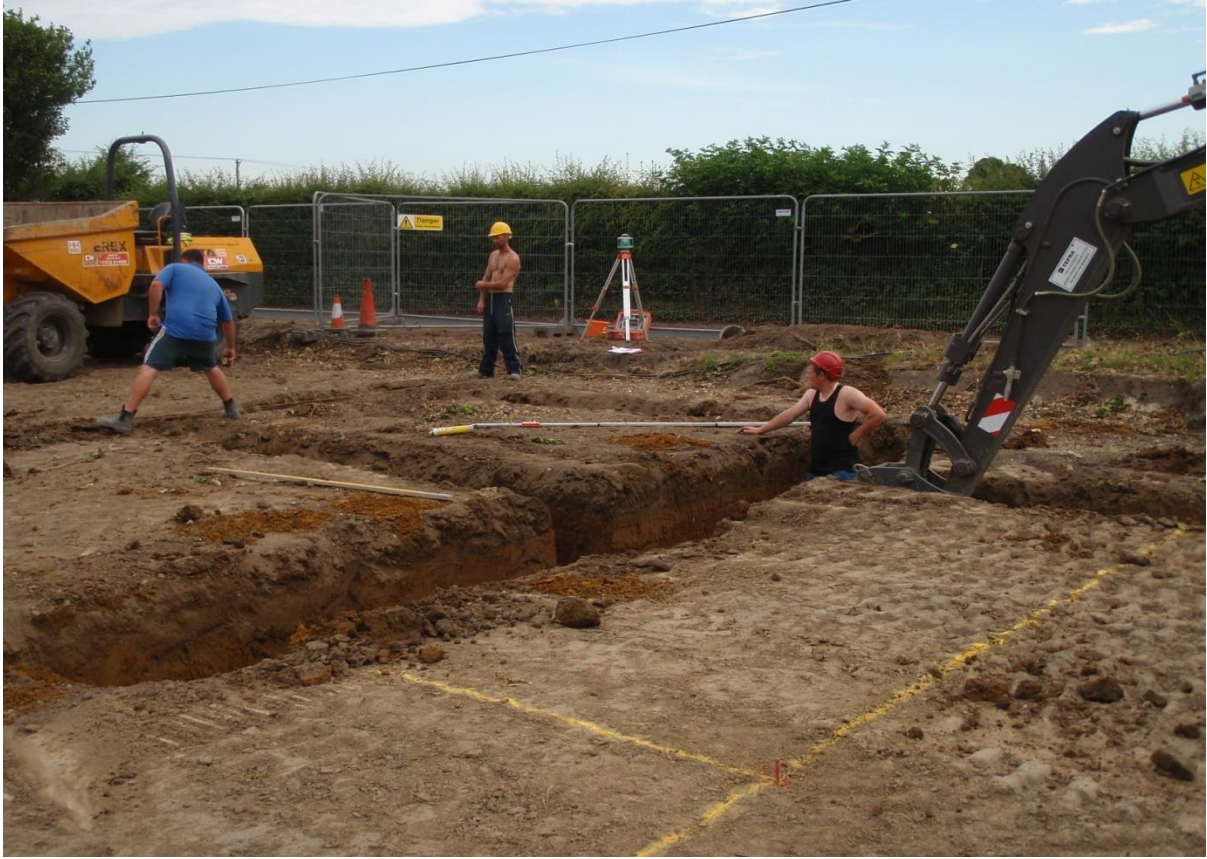
Plate 5. Cutting foundations Plot 6
