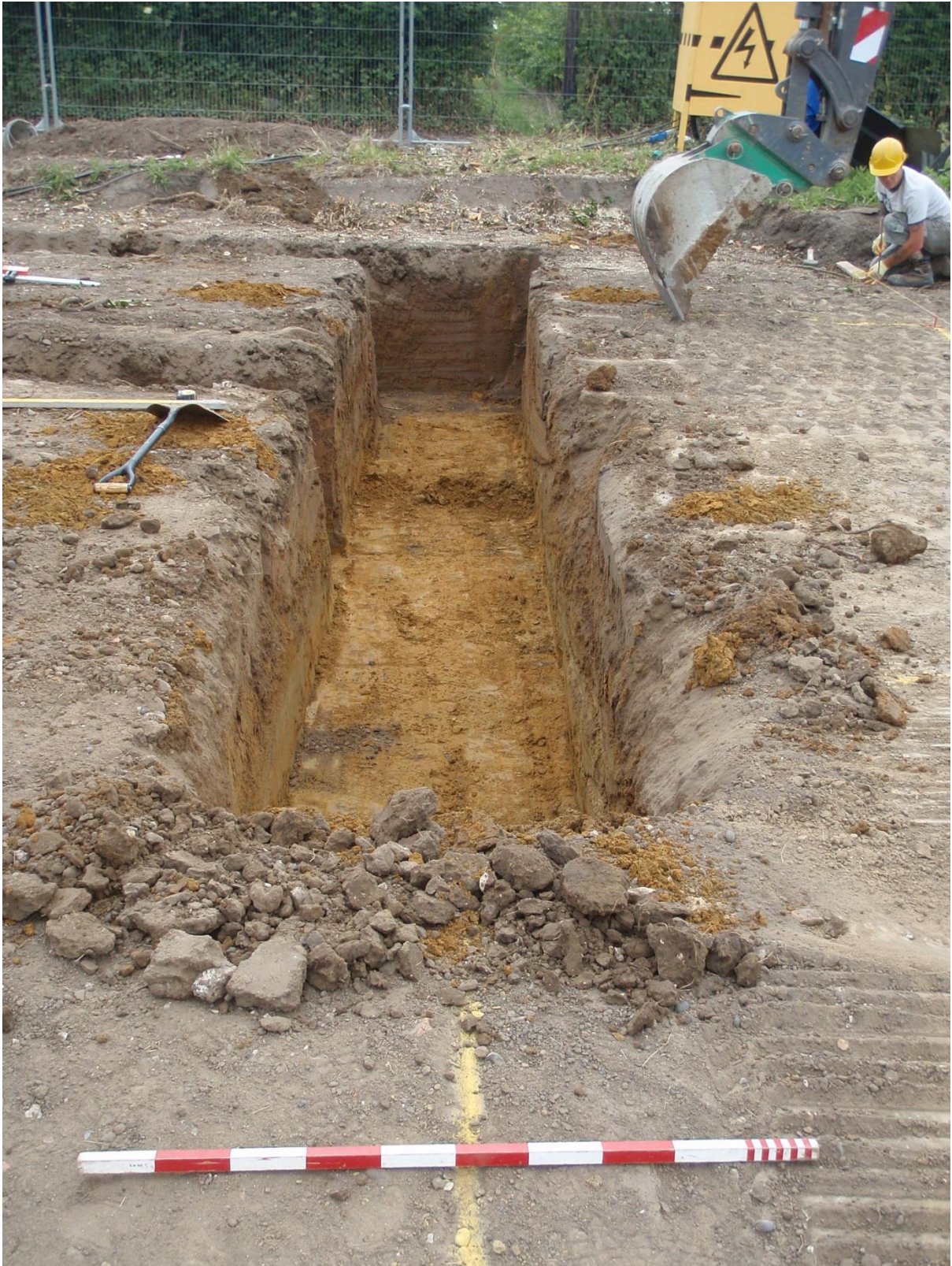
Plate 9. Cutting foundations Plot 5
