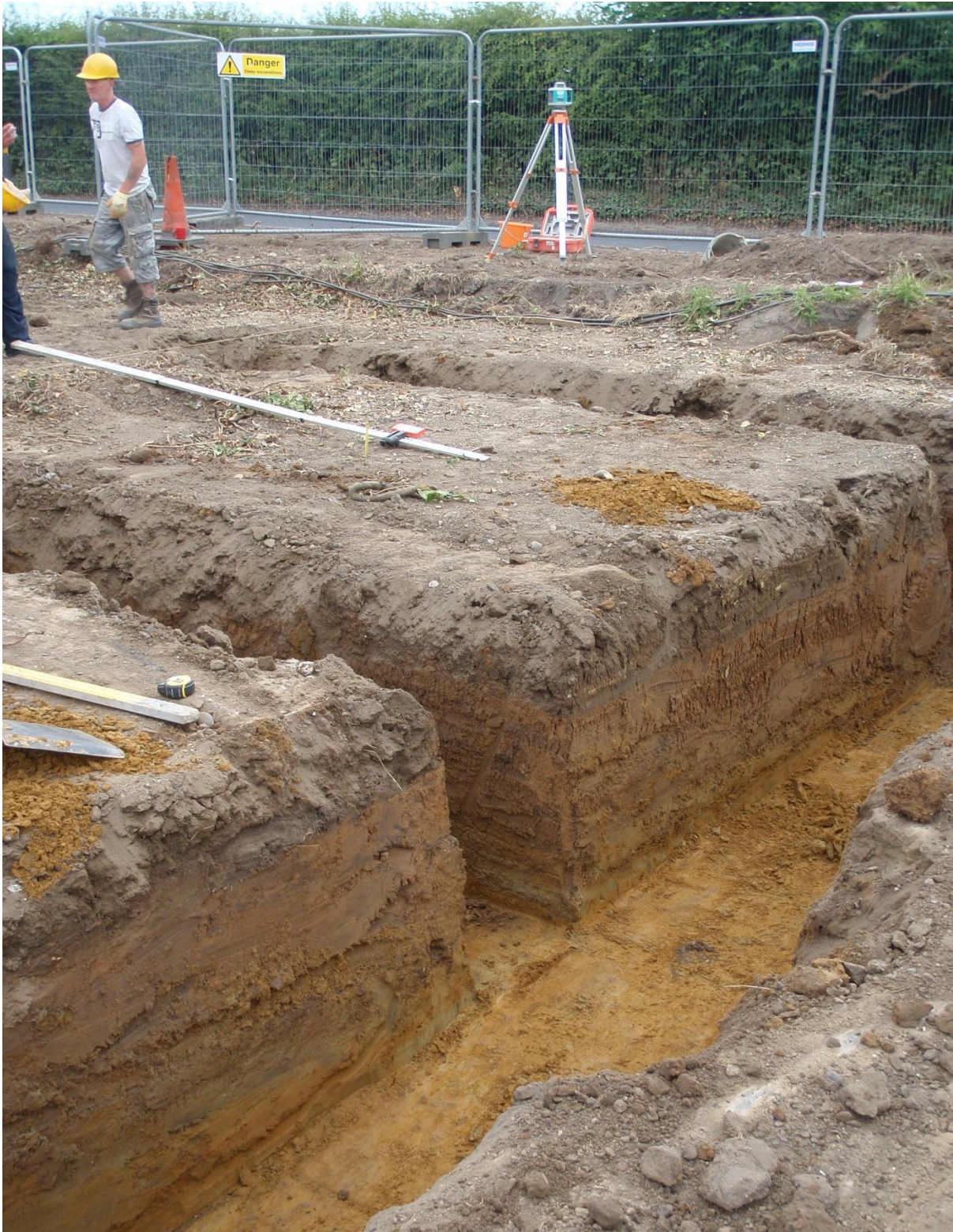
Plate 10. Cutting foundations Plot 5
