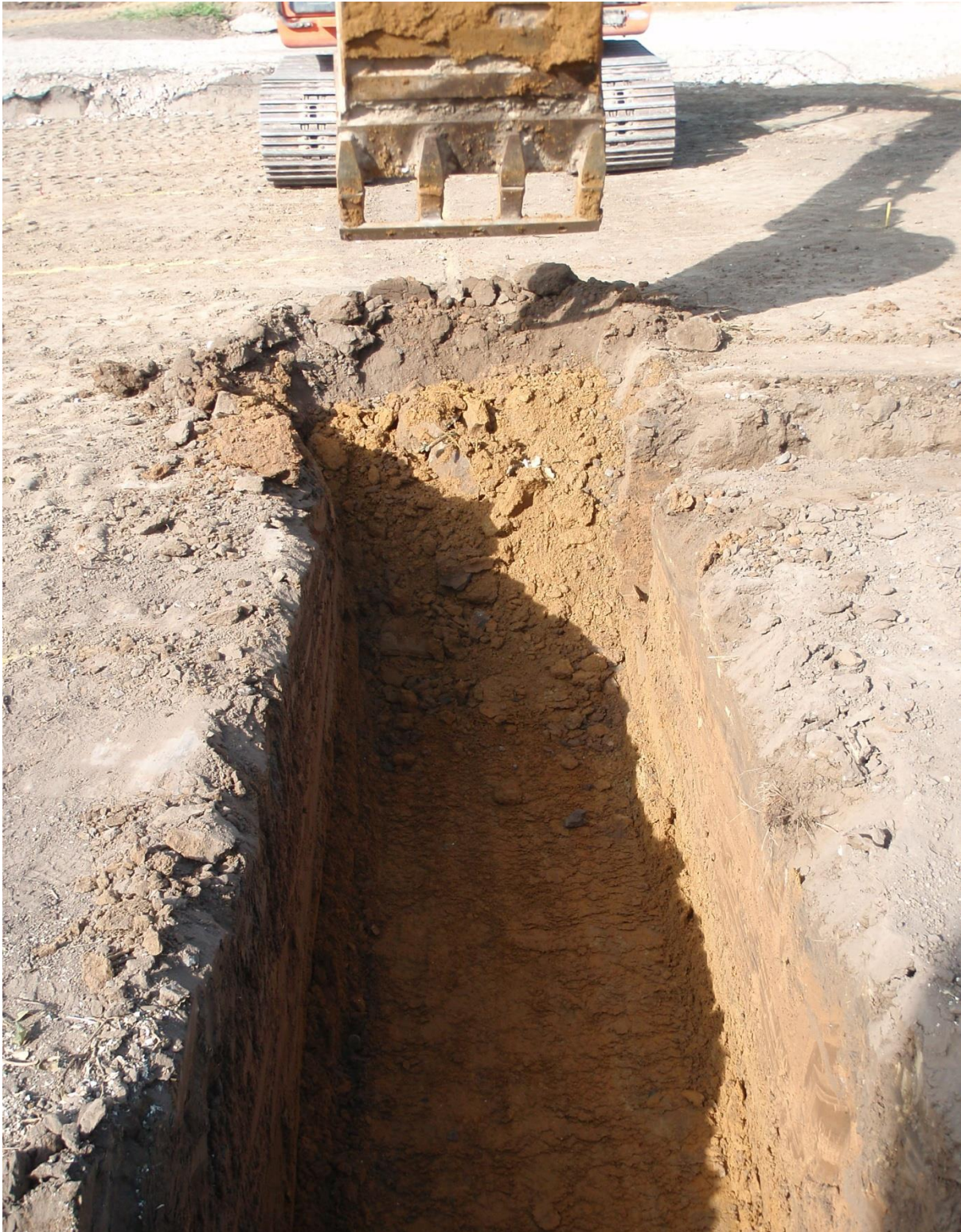
Plate 11. Cutting foundations Plot 2
