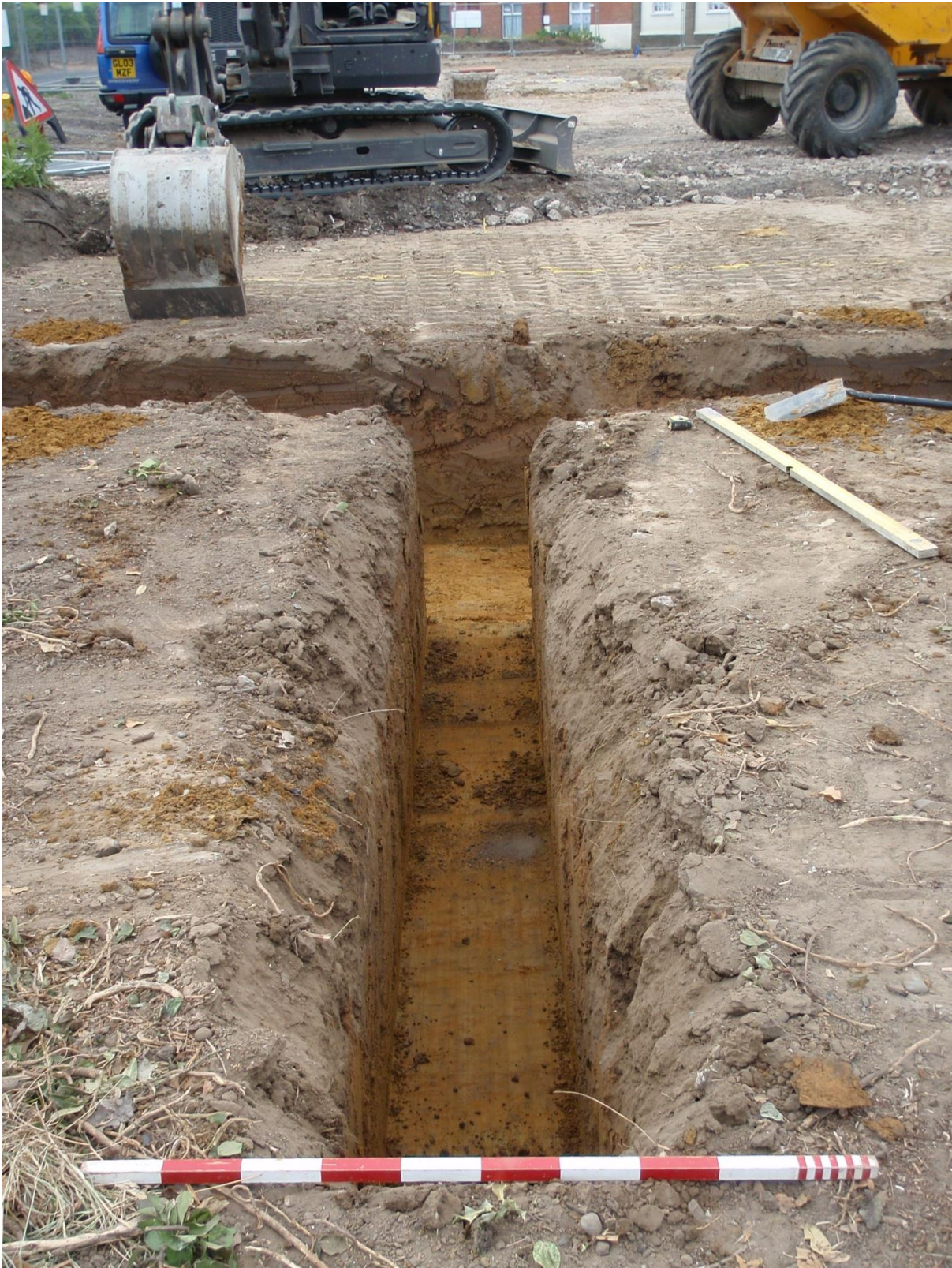
Plate 7. Cutting foundations Plot 10
