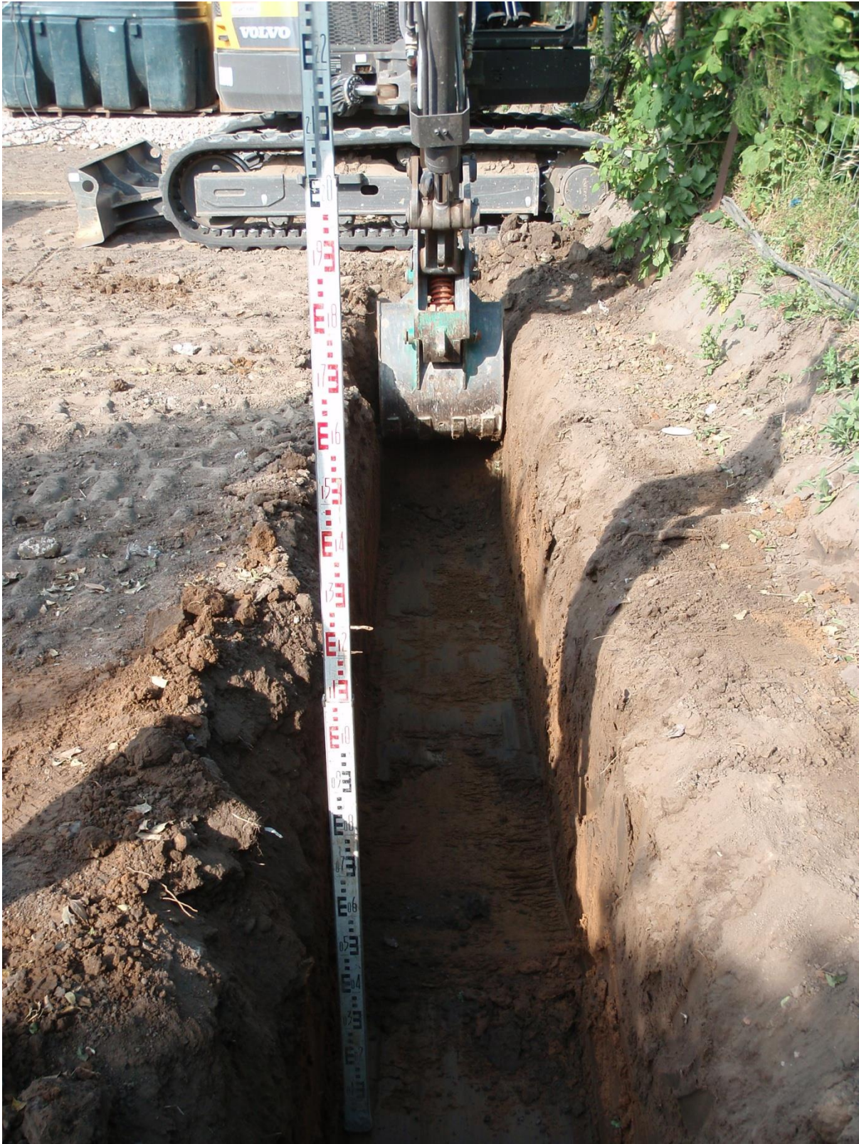
Plate 4. Cutting foundations Plot 8
